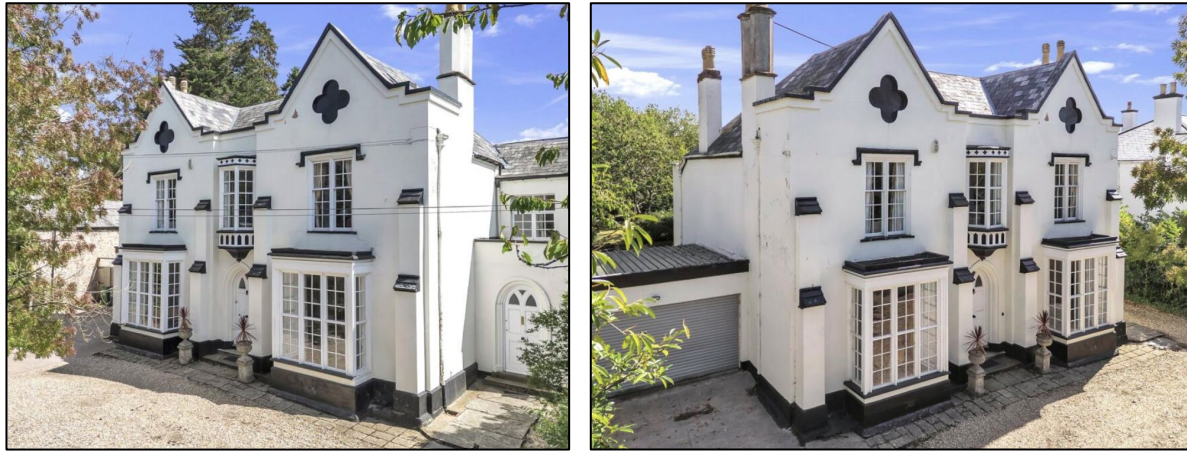
Burwood Principal Gothic Elevation following roof repairs
